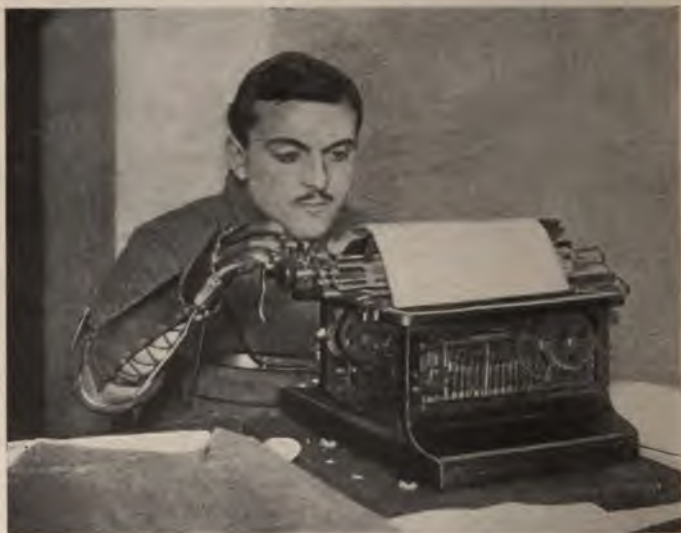
FIG. 12.—Amar arm used in typewriting.
